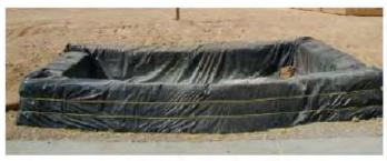
Line concrete/contaminate washout areas with impervious material like plastic. Maintain and periodically remove hardened soils.
