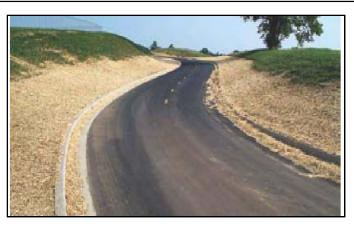
Very good treatment of roadside areas with blown straw after seeding. In areas near lakes, streams, and rivers, straw in roadway must be cleaned up after application.
