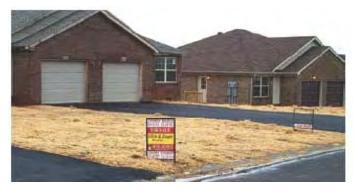
Excellent application of hand scattered straw mulch in new residential subdivision. Work sites must be seeded and mulched as soon as final grade is established. Crimp mulch into soil with dozer tracking or disk harrows set straight to prevent straw from blowing.
